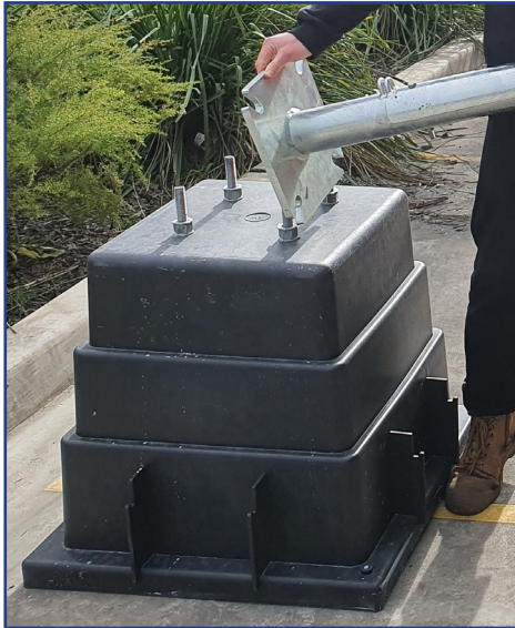
Fig. 2.3a Mounting pole onto concrete base
