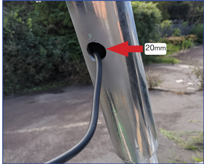
Fig. 2.4a Solar panel power cable hole location
