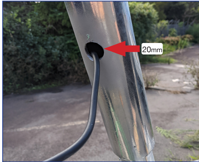
Fig. 2.4a Solar panel power cable hole location
