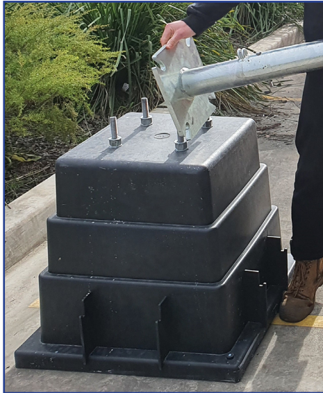
Fig. 2.3a Mounting pole onto concrete base
