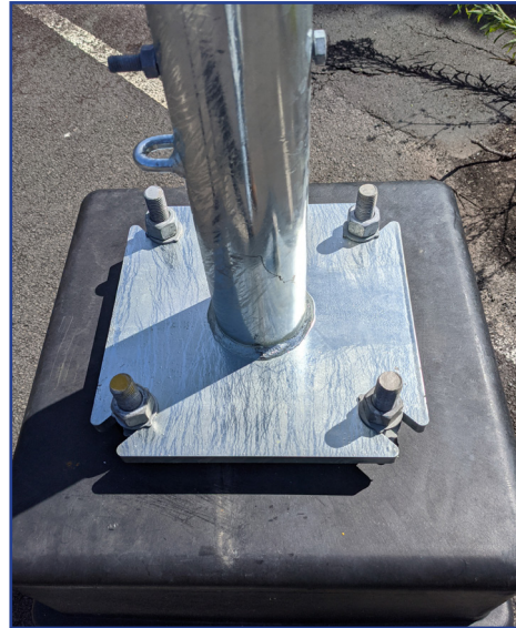
Fig. 2.3b Pole fixed onto on concrete base
