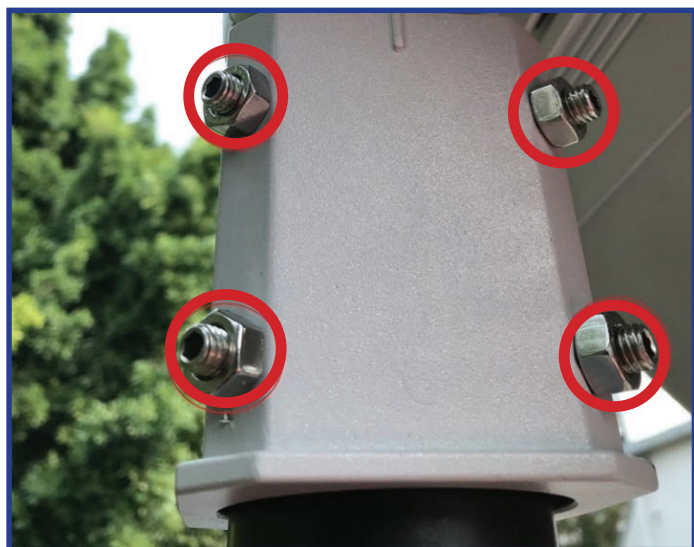
Fig. 2.1b Installed grub screws
